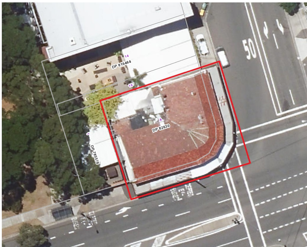
Figure 1: Property containing the Alexandria Hotel (Image: SIX maps)
