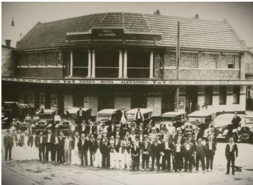
Figure 13 The Alexandria Hotel photographed not long after completion. The stepped parapet above the balcony was removed during or after the second half of the 1980s. It contained the name of the hotel, reflecting a common practice of the 1930s. Source: http://www.alexandriahotel.com.au/history.aspx
