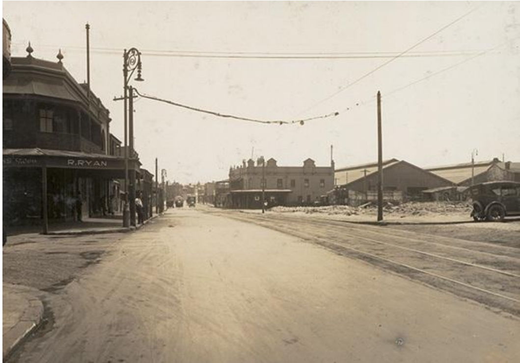
Figure 6 Demolition along the northern side of Henderson Road between Wyndham and Garden Streets, 23 November 1927. The Alexandria Hotel can be seen in the centre of the photograph and is yet to be demolished.
